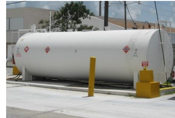
10,000 Gallon Diesel Double-Wall Steel AST
