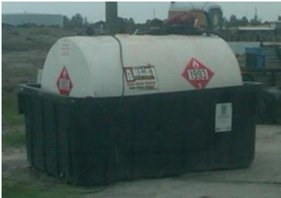
Single-Wall Steel AST in Plastic Containment
