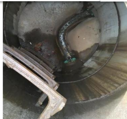
Manhole MS3 inlet photo.
